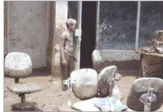
The library at Northern University Nowshera was completely destroyed.
