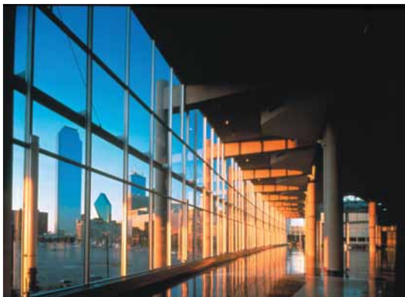
A curtain window wall frames expansive views of the city skyline at the Dallas Convention Center.
